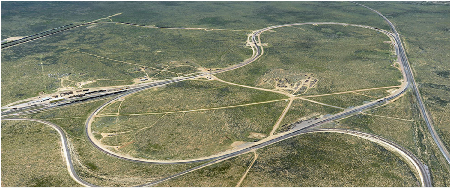
Transportation Technology Center i Pueblo, Colorado, from above
